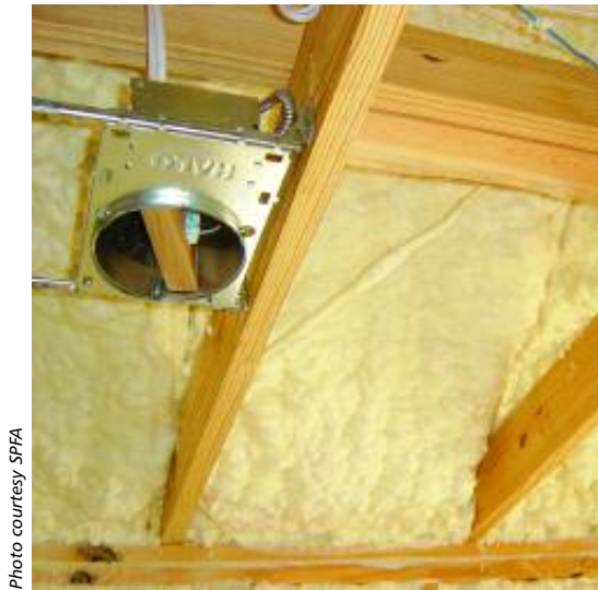
SPF forms a seamless layer of insulation and offers the potential for impressive energy savings.
